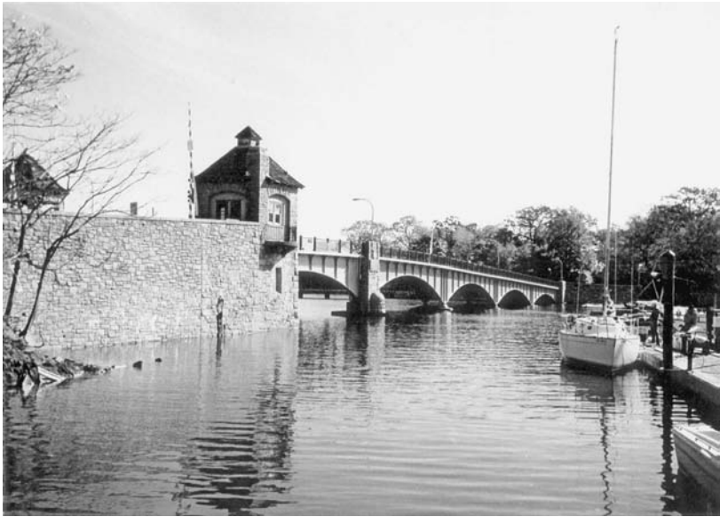
FIGURE 7.5 Protective coating on a bridge. (Courtesy of 21st Century Coatings, Inc.)
