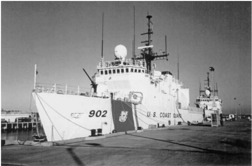
FIGURE 7.4 Exterior protective coating on a Coast Guard ship. (Courtesy of 21st Century Coatings, Inc.)
