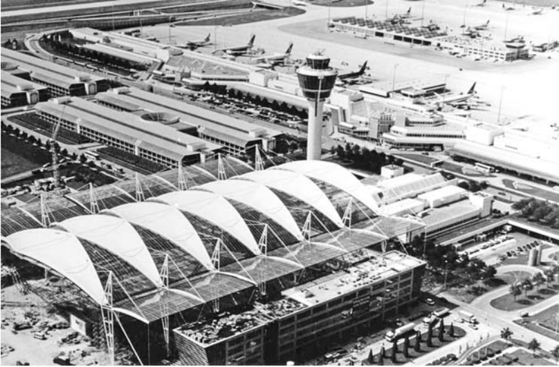
FIGURE 6.7 PTFE roofing elements at the Munich Airport Center. (Courtesy of Skyspan Europe GmbH.)
